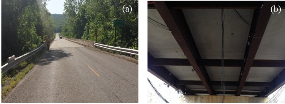
Figure 4.1. (a) Road view and (b) underside of bridge (Photo by author)
